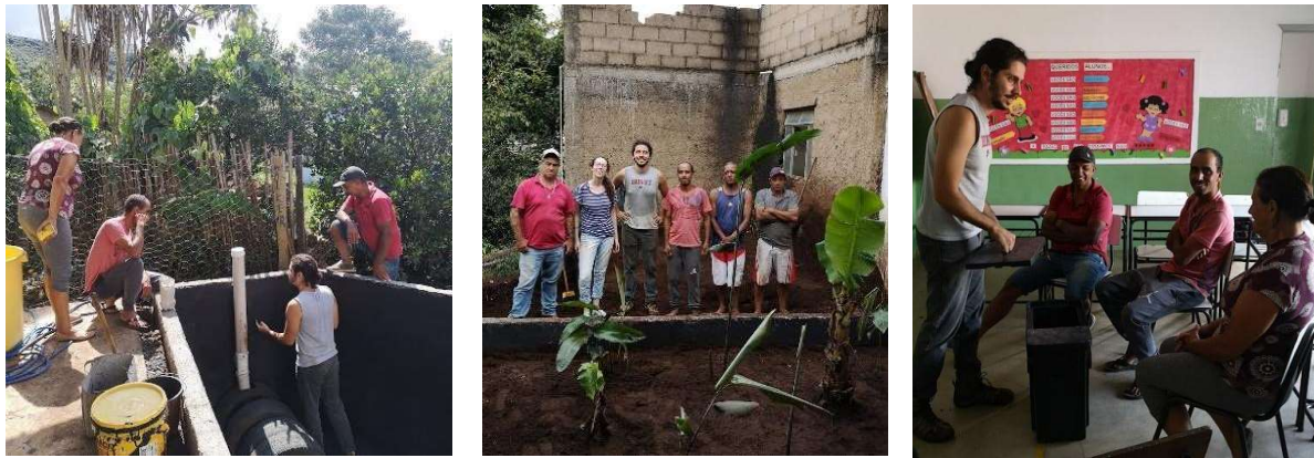
Figure 6: records of the participative construction of TEvap with the community.
